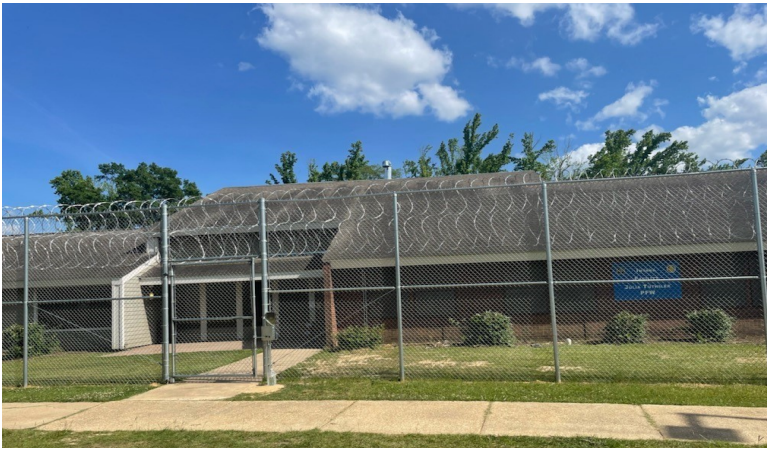
Tutwiler Quarantine Intake with new perimeter fence
