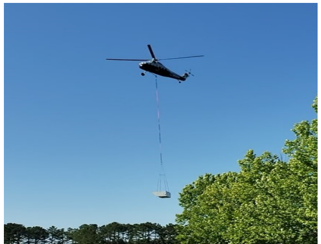
A helicopter suspending several HVAC units for strategic placement on the facility's roof.
